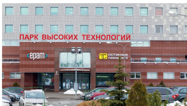
Building complex of the High Technologies Park. Business incubator of High Technologies Park and the office of EPAM. Belarus, Minsk, January 2017. Image source: ElROI / Shutterstock.com.
